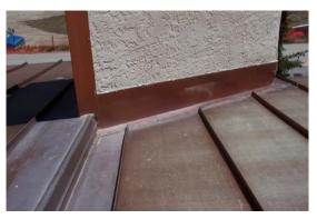
roof leaks. The metal roof panels and underlayment would need to be removed and damaged sheathing replaced.
