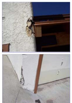
Replacing the stucco with an alternative cladding system is also an option. A stone, or a faux stone, may work well. If choosing a stone façade we recommend full depth mortar joints. Open joints at higher elevations are prone to damage from the dramatic freeze thaw cycles.
