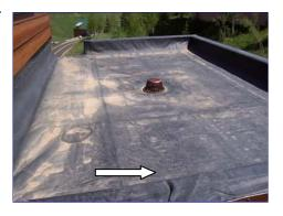
**Recommendations:** The membranes were in good condition for their age. We did note that the adjacent parapet walls did not have a parapet caps and were just wrapped with the EPDM membrane. These metal parapet wall caps are required by the manufacturer. We recommend installing the flashing if the membrane starts to prematurely deteriorate. The roofs should last another 12 to 14 more years.
