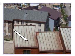
We observed damage to stucco and siding from ice/snow fall from the roofs. The eaves on the buildings have no overhang relative to the vertical façade. We received report of ice damming problems during the winter months.
