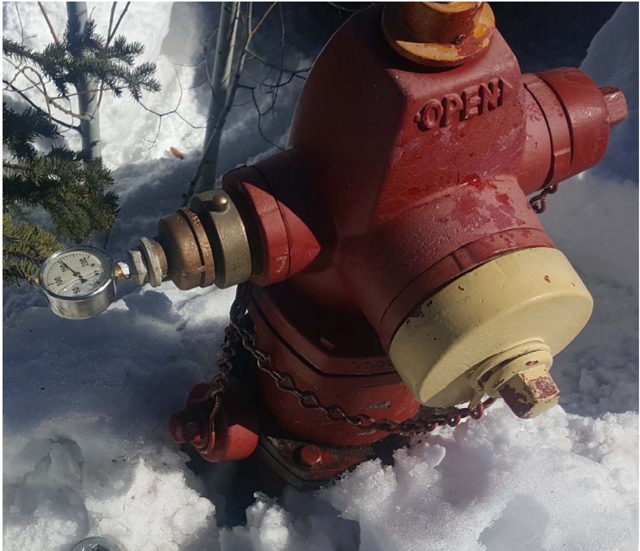
Fire Hydrant With Pressure Gauge - Post Repair
